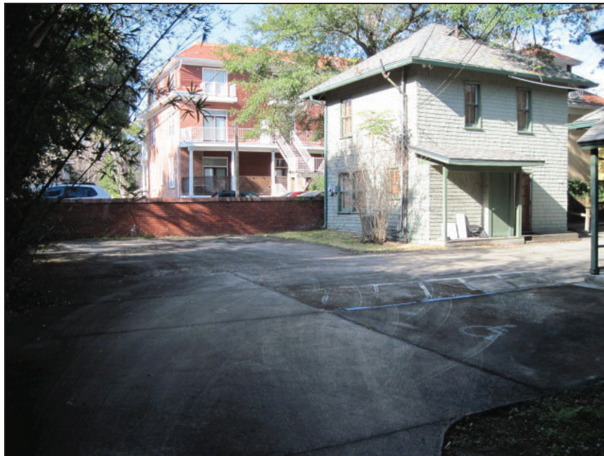
Rear parking area, wall, and 2-story apartment structure.
